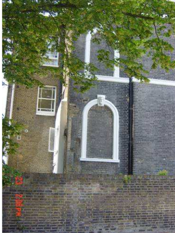
Figure 20: two blind windows on a flank elevation to Shooters Hill Road
