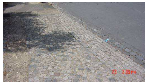
Fig 41: low pitched slate roofs Fig 42: Traditional setts for gully and crossover in Hervey Road
