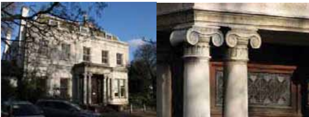
South elevation and detail of columned porch
