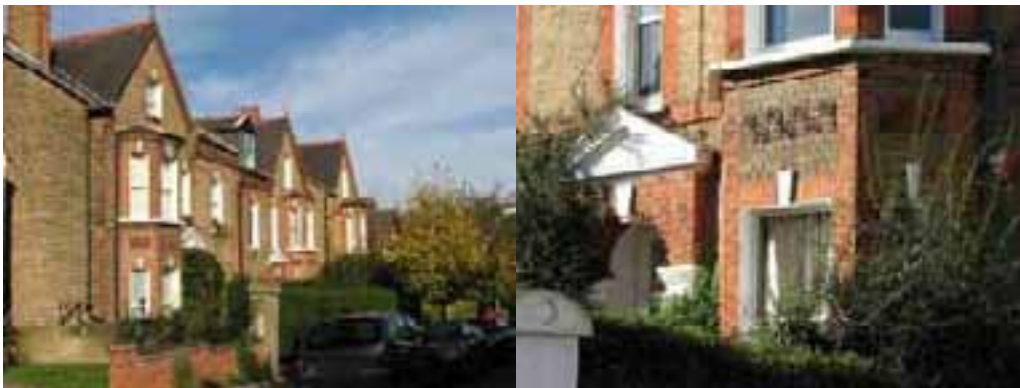
74-78 Foyle Road, Locally Listed Buildings
