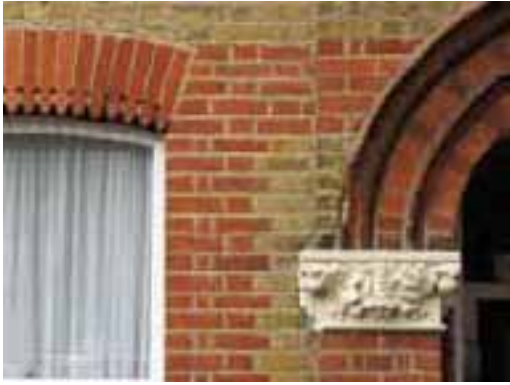
No. 49, detail showing fine gauged brickwork
