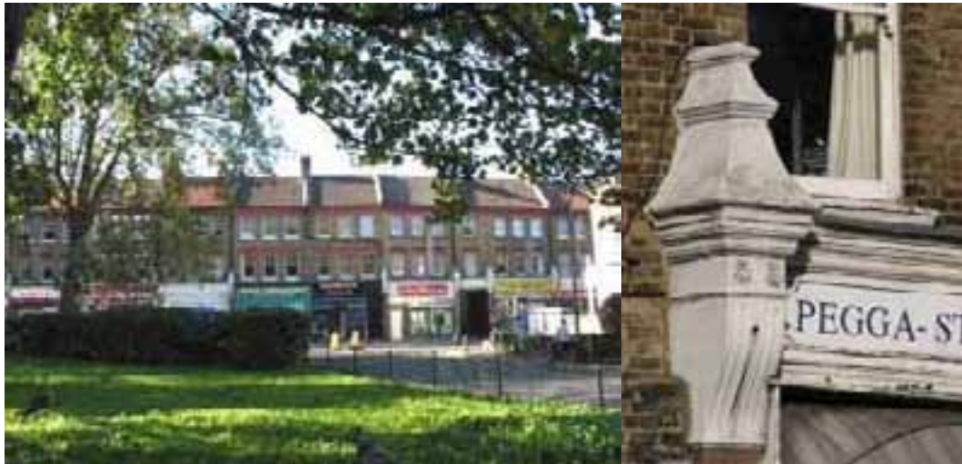
Westcombe Hill shopfronts with example of surviving console bracket and moulded fascia
