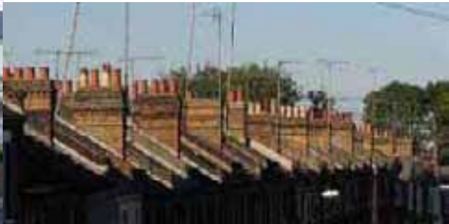
Deep brick chimneys
