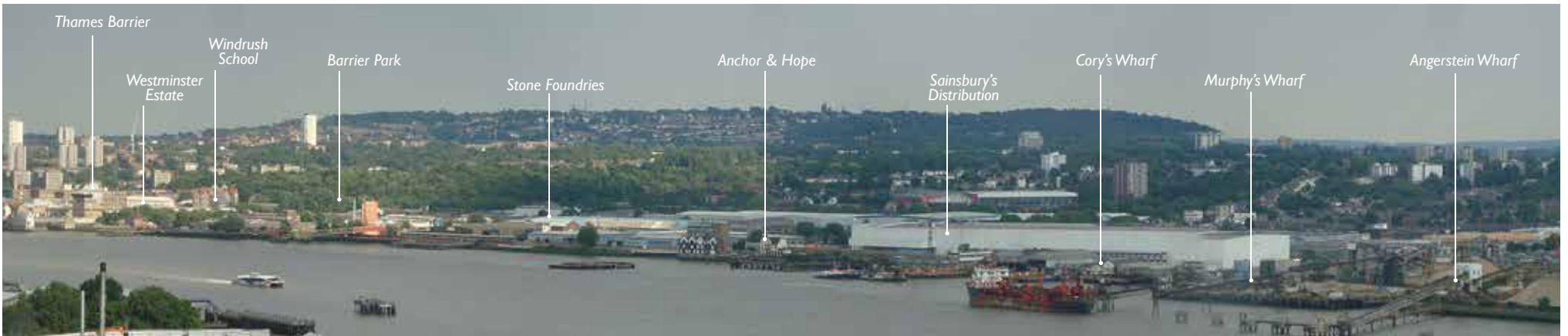
Panorama showing Charlton Riverside site, viewed from the north west, with key taller buildings and structures identified
