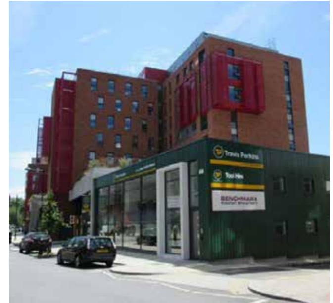
Travis Perkins, with student accommodation above (Camden)
