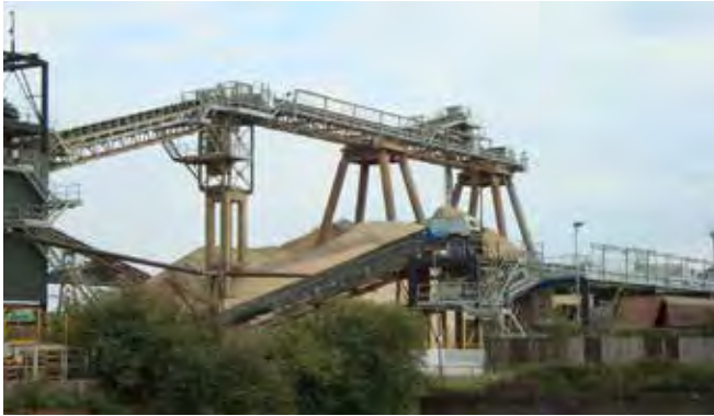
Aggregates industry plant and structures
