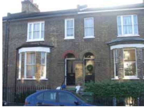
Figure 34: Devonshire Drive houses
