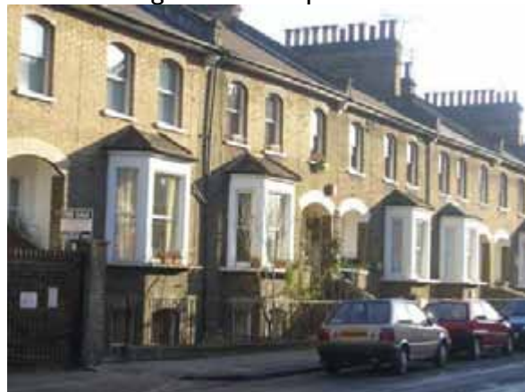
Figure 58: Langdale Road: east side
