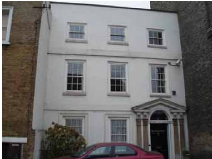
Figure 24: Wellington House - Listed Grade II
