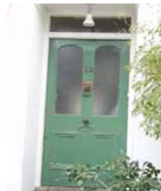
Figure 42: Door in Egerton Drive
