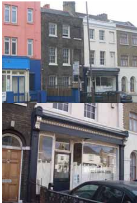
Fig 63: South side of Blackheath Road 70-80 Fig 64: fine original Edwardian shopfront – no 72
