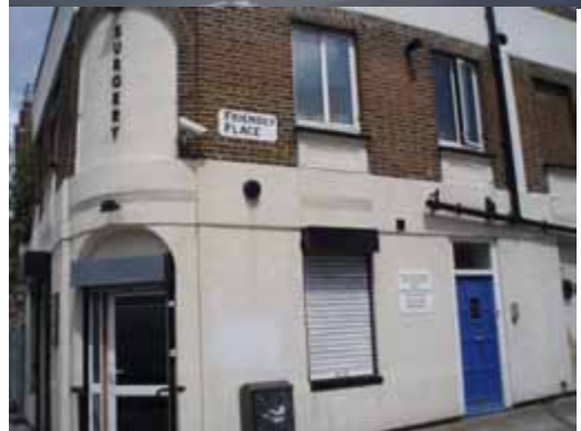
Figure 51 & Figure 52: Lewisham Road and Friendly Place: One building has been demolished, the building on the right (9 Lewisham Road) is Listed mainly for a shopfront which appears to have been removed some time ago.
