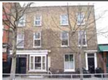
Figure 21 & Figure 22: 133-135 GHR - a pair of unlisted but Listable early 19 th century Georgian townhouses, plain and restrained style. 131 having been altered externally probably in late 19 th century to create a ground floor shop and side doors to residential accommodation above. 131 has window replacement, and is in the worse condition - but is worth inclusion especially as it has group value with no 135.
