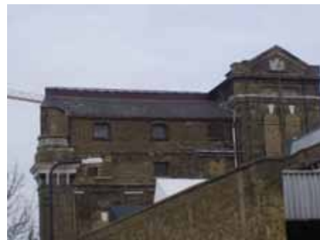
Figure 32: Davy's Wine Vaults - warehouse at rear, former Lovibonds Brewery Figure 33: Close up showing large pillar on left of building with base of secondary plinth above. This photo suggest that when a Brewery this was a large chimney, which it seems may have later been truncated when the building was converted to a store
