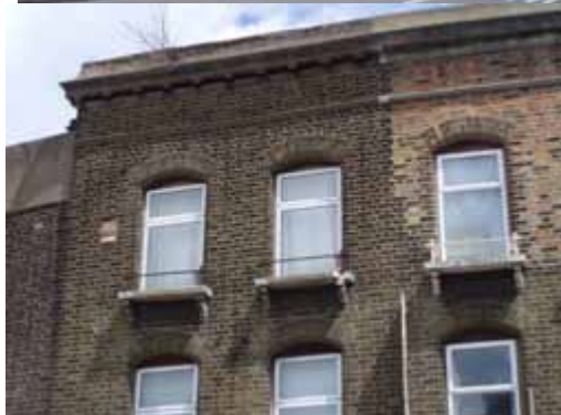
Figure 55: 29-33 Lewisham Road: late Victorian Parade with surviving shop-front pilasters Figure 56: 29-31 Lewisham Road - detail shows dentil brick cornice, brick string course, arched window headers, and disfiguring replacement windows
