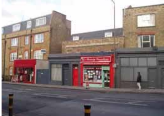
Figure 57 Mixed 19 th c. Buildings Blackheath Road
