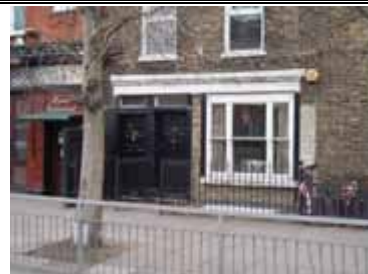
Figure 21 & Figure 22: 133-135 GHR - a pair of unlisted but Listable early 19 th century Georgian townhouses, plain and restrained style. 131 having been altered externally probably in late 19 th century to create a ground floor shop and side doors to residential accommodation above. 131 has window replacement, and is in the worse condition - but is worth inclusion especially as it has group value with no 135.
