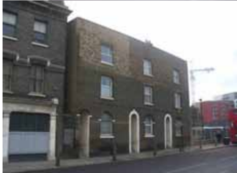
Figure 7: Inner side of Greenwich High Road - School at No 2 Figure 8: Inner side of Greenwich High Road - very early plain austere houses at nos 20 - 24
