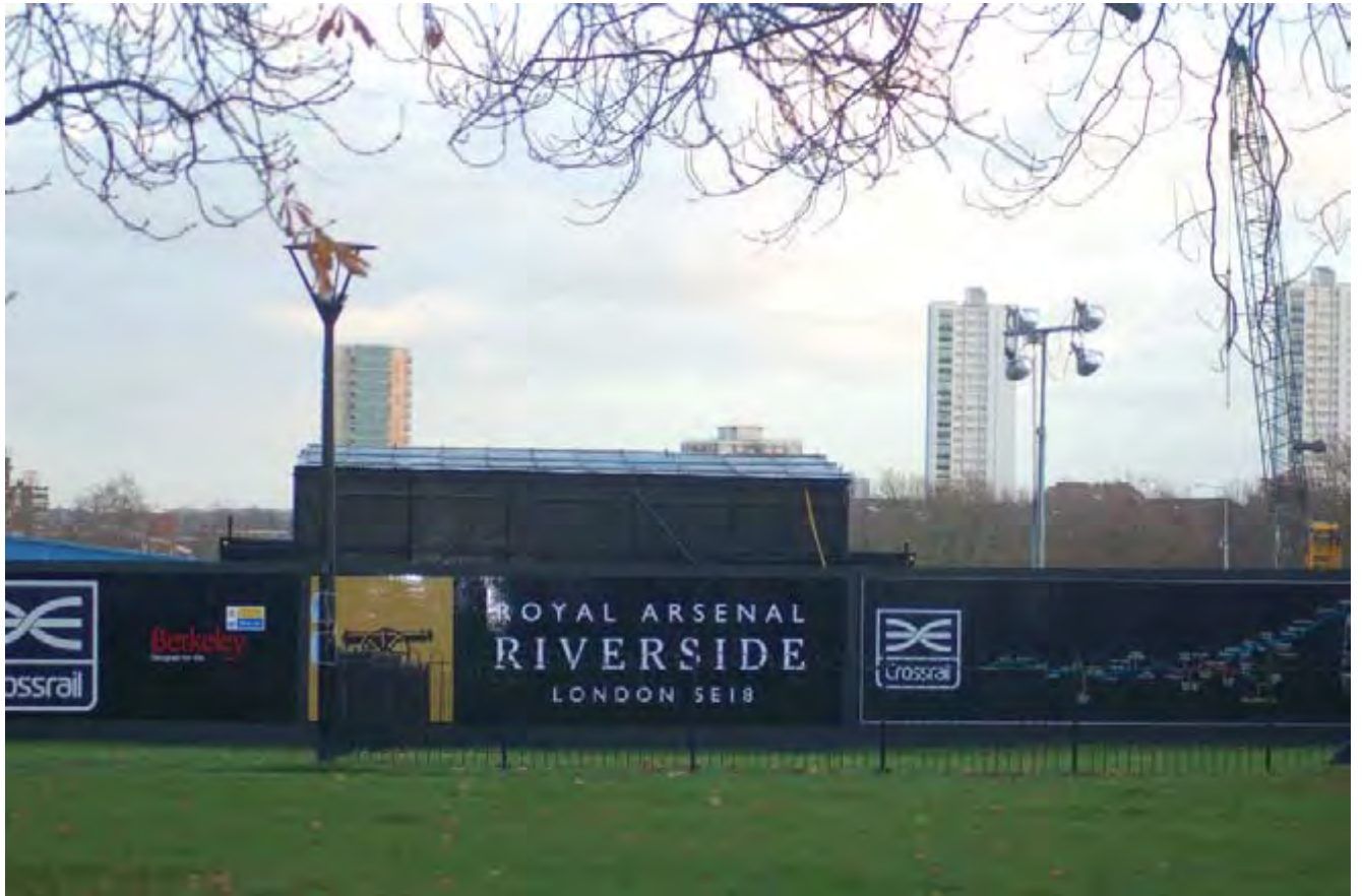
Woolwich Crossrail on site December 2011
