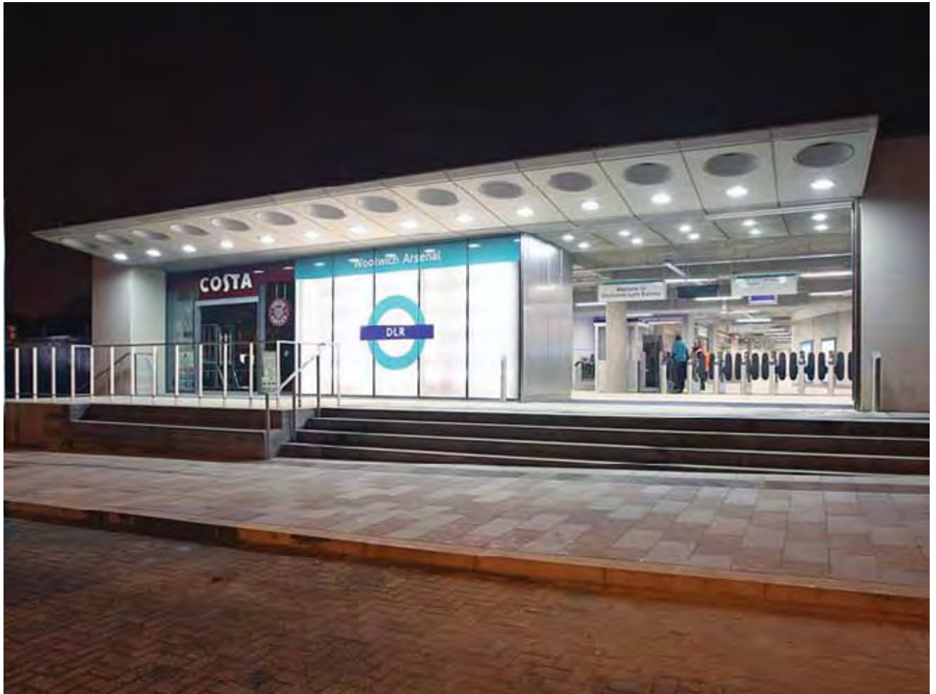
The recently completed Woolwich Arsenal DLR
