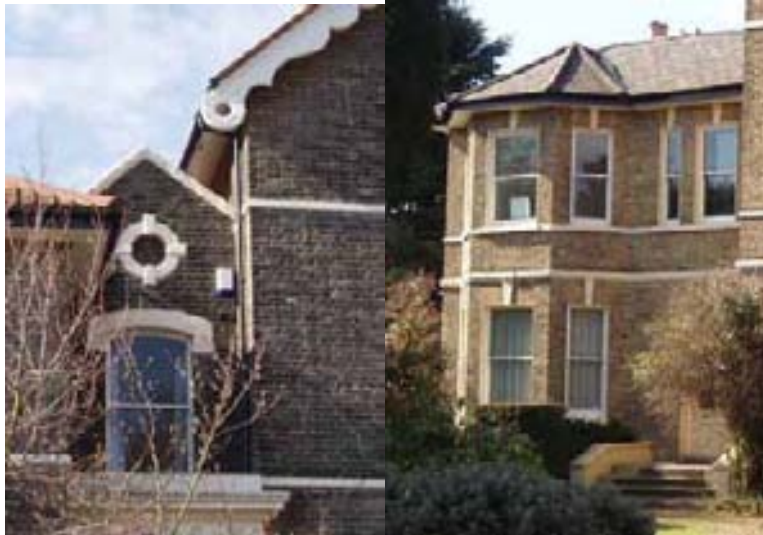
Decorative barge-board and blind circular window at no. 46 Projecting keystones at no. 50
