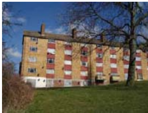
Middle Park Avenue nos. 553-639, built 1958-9 by Woolwich Borough Council
