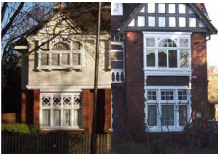
Unusual glazing at nos. 87 and 95
