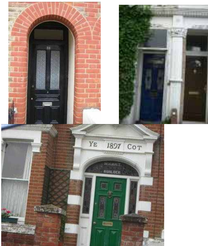
Fig 92: Quality restoration – old door set in recessed porch; Fig 93: Two doors, one old, one new; Fig 94: Elaborate 1897 door
