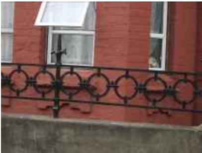
Figure 95: Interesting newly reinstated ornamental railings in front of unsightly painted bricks
