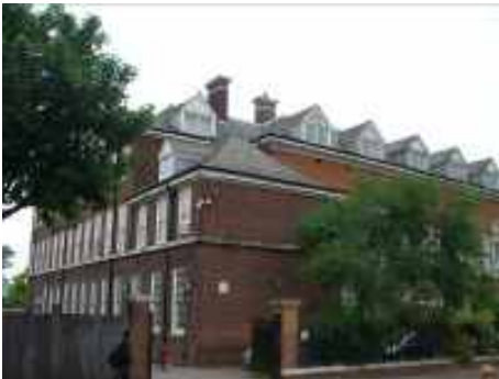
Figure 71: Plumstead Manor School Road
