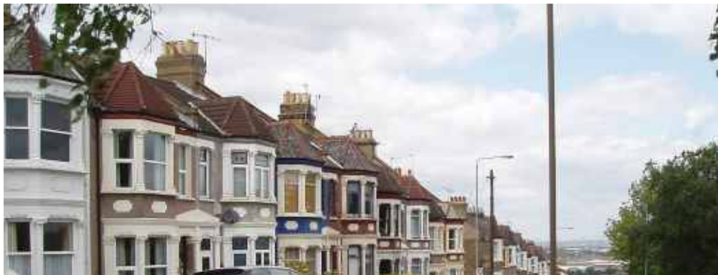
Figure 62: typical bay fronted late Victorian housing – Lakedale Road
