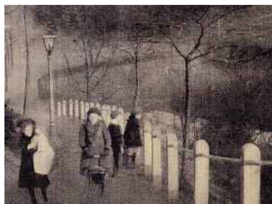
Figure 101: c. 1906 post and rail boundary treatment (at bottom of The Steps) – source old postcard
