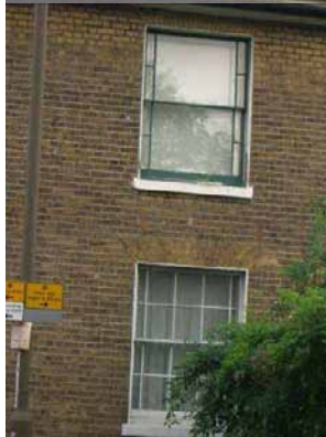
Figure 48: Unity cottages margin light windows
