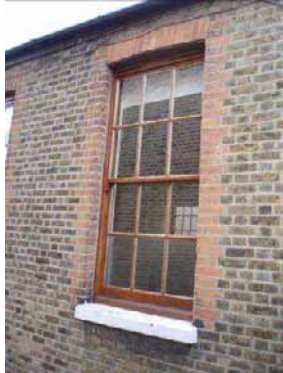
Figure 45, Figure 46, Figure 47: 1865 well preserved Brethren Chapel 13 Plum Lane with sliding sashes
