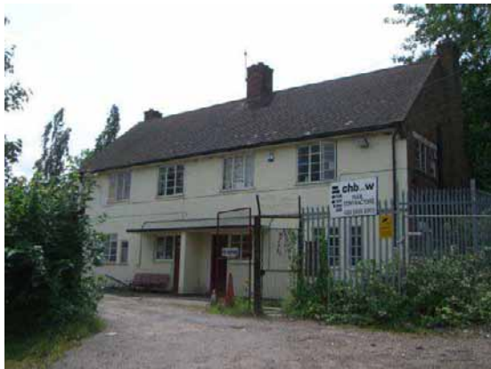
Figure 36: cottages at north end of Rockliffe Gardens
