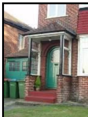
Original open porch design, in Plum Lane
