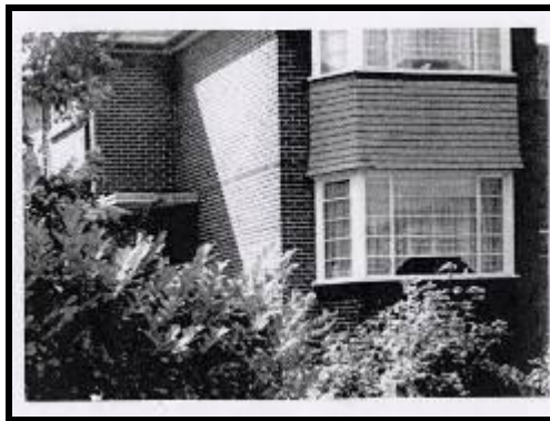
An old photograph of canted bay with steel windows at 26 Ashridge Crescent
