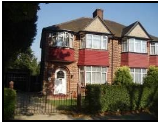
Eskdale semi – note Oriel bays, gables, and clay tiled roofs, the windows have been replaced with good replicas
