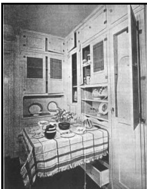
Laing's De luxe kitchen – taken from sales leaflet. The “table” is a fold out from the cupboard. The ventilated larder can just be seen above it to the right of the corner. The fold down ironing board can be seen in the cupboard pointing upwards at top right.
