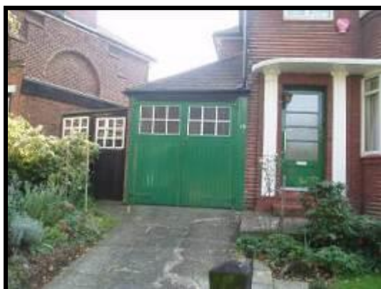
Original garage doors with surviving side garden gate
