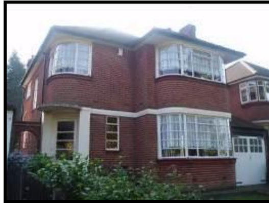
Olympia detached – for construction reasons this could only be built with Jubilee front
