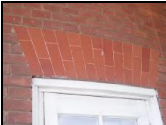
Fine gauged brick with lime pointing
