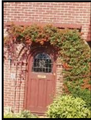
A quality replacement door, set with triple arched and dentilled surround There is also a good double-arched dentilled surround at 31 Ashridge
