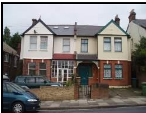
Semi detached pair – Eaglesfield Road. Both houses have lost their front gardens to off street parking. The house on the left has inserted roof lights, but retains the original upper windows. That on the right retains its porch.
