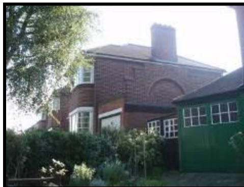
Belford Jubilee detached – notice depth of house, the expressed external chimney was only built on detached units
