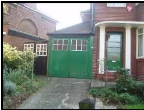
Jubilee art deco 4 light front door – notice original side garage and unequal lights on front door to align the glazing bars with those of the original bay windows (now replaced)
