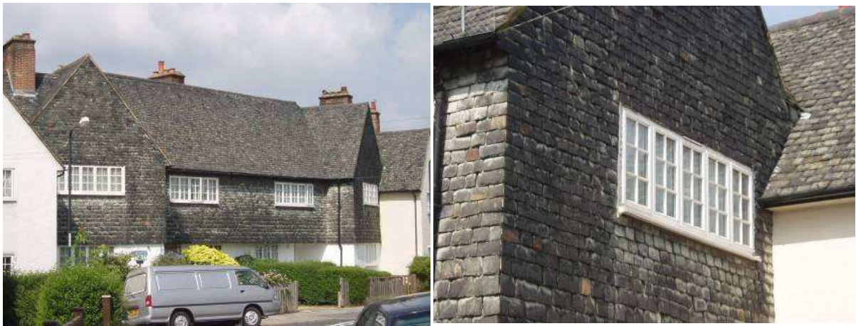
Figure 26: extensive use of fine Westmoreland roof and hung slates
