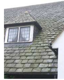
Fig 39: rear of house showing relayed Westmoreland slates – with central band of good Welsh slates
