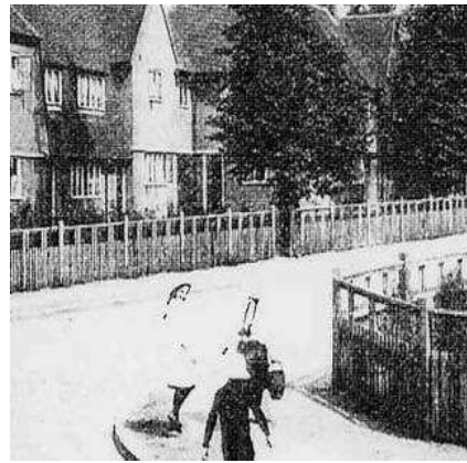
Fig 43: 1915 photo showing original fence in Dickson Road;
