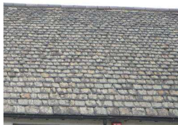
Figure 35: fine slate laying in diminishing courses; Figure 36: fine slate laying in diminishing courses
