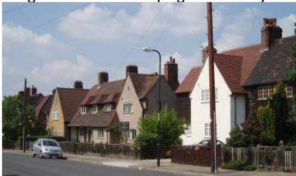
Fig 51: Original front dormers at first floor level on Downman Road – with hipped and pitched capping roofs.
