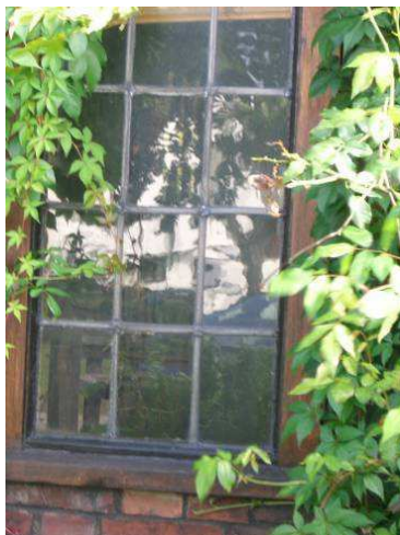
Figure 31: original leaded Lights in steel windows set in wood frames.
