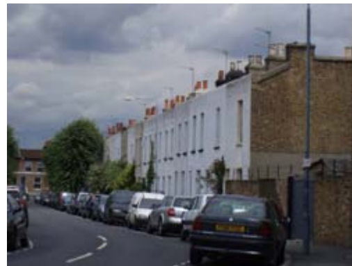
Figure 14: Old parapet fronted cottages Bowater Place
