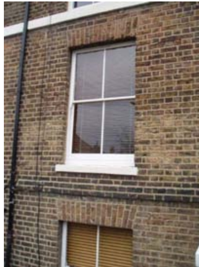
Figure 59: Characteristic mixed stocks and traditional sash windows
