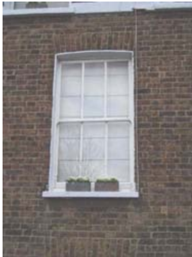
Figure 55: Georgian small pane windows
