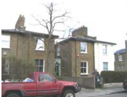
Figure 16: 1840's semi detached villas 101-7 Old Dover Road
