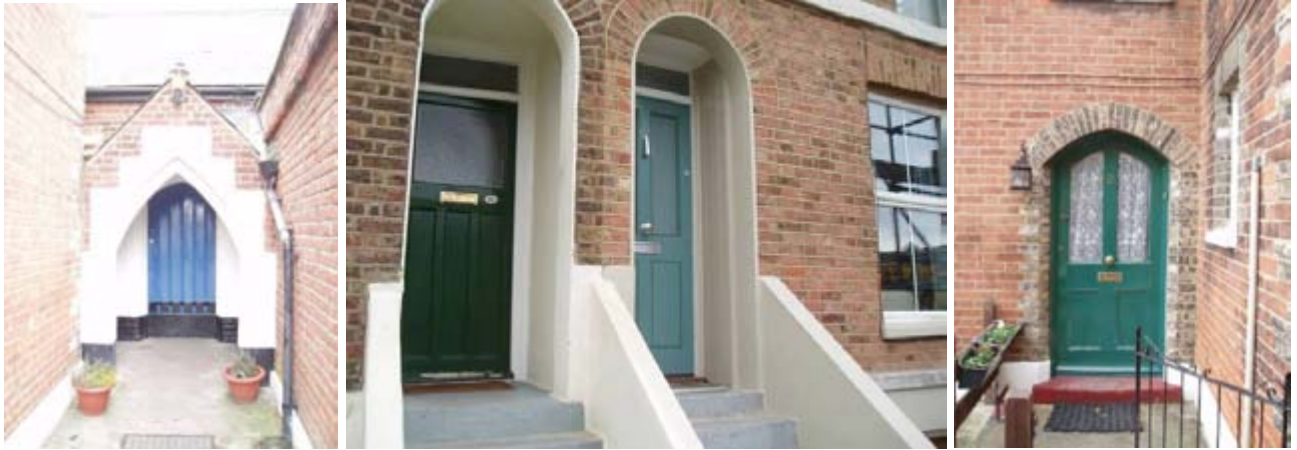
Figure 52 53 & 54: some local doorways and doors
