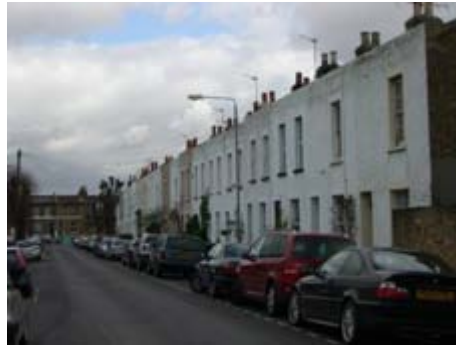
Fig 48: Bowater Place – older parapet fronted houses
