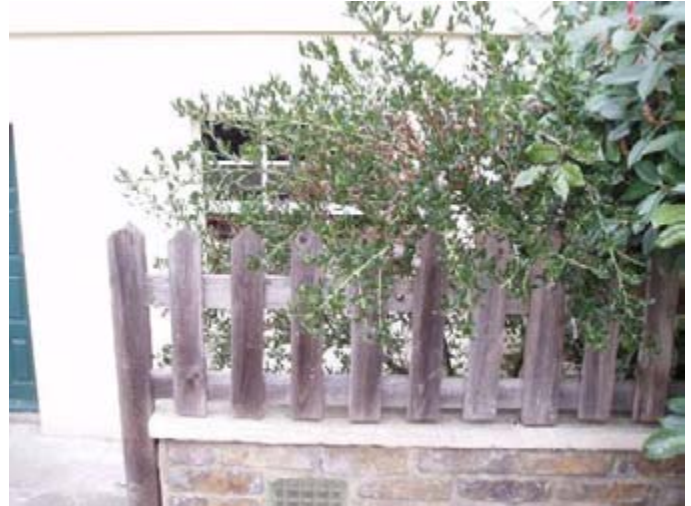
Figure 56: front boundary fence
