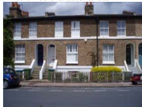
Figure 17: Stylish mid-Victorian terraces with exaggerated eaves, yellow stocks, red brick dressed door arches, recessed porches, external entrance stairs picket fences small pane Georgian windows and semi basements
