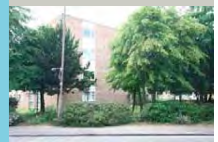
Rear of Wycombe Court
