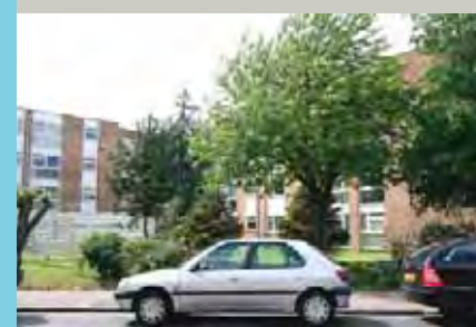
Rear of Wycombe Court
