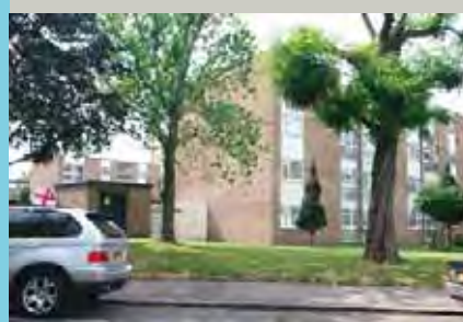
Rear of Wycombe Court
