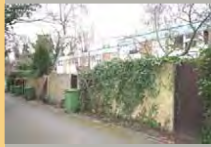
Rear of Corner Green
