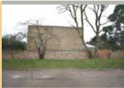
Wall, side of 15 Morden Road
