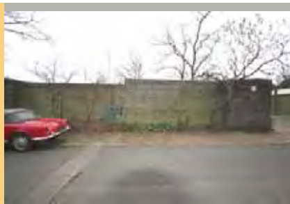
Wall between garage blocks
