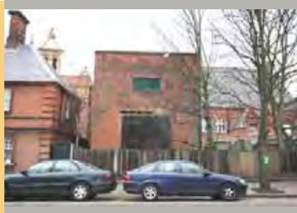
Redundant transformer station
