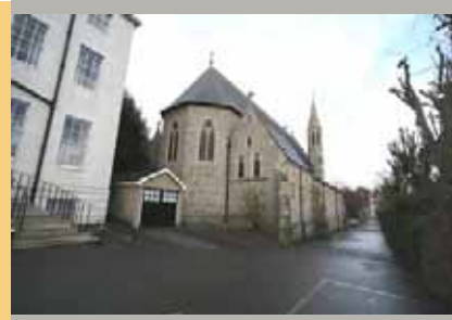
Rear of Church
