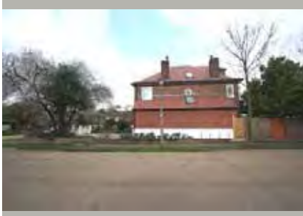
Garage to rear of 37 Foxes Dale
