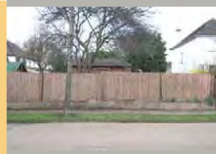
Building to the rear of 37 Foxes Dale
