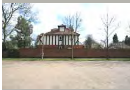
Side of 52 Brooklands Park
