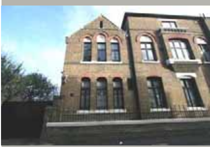
Apartment block (former school)
