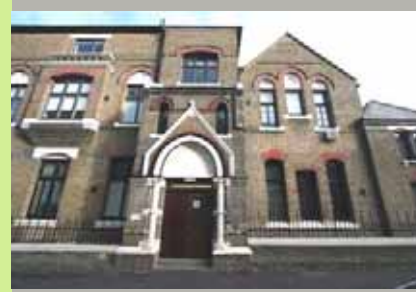
Apartment block (former school)
