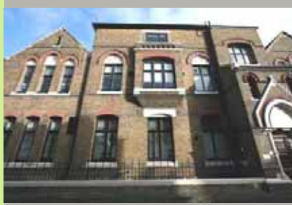
Apartment block (former school)
