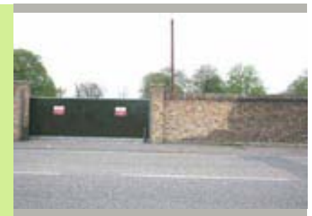
Listed wall and gates
