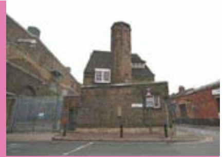
Disused Power Station
