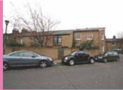
Rear of buildings
