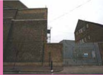
Disused Power Station
