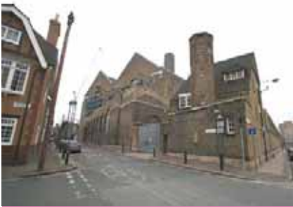
Disused Power Station
