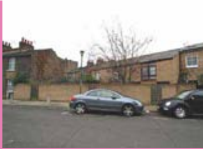
Rear of buildings
