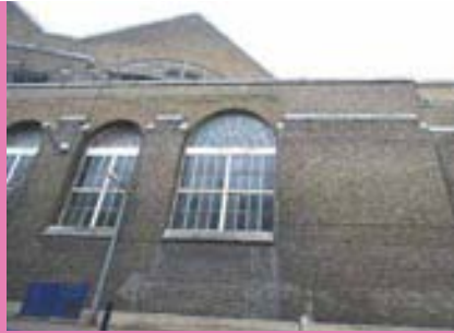
Disused Power Station
