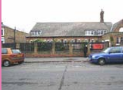
East Greenwich Community Centre
