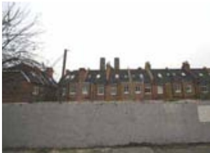
Rear of Trenchard Street
