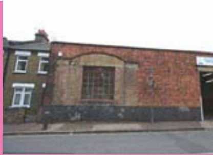
Park Row Garage
