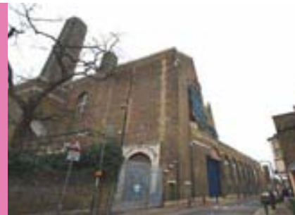
Disused Power Station
