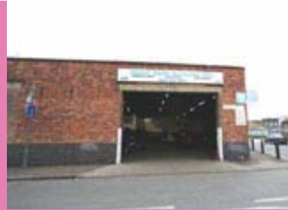
Park Row Garage
