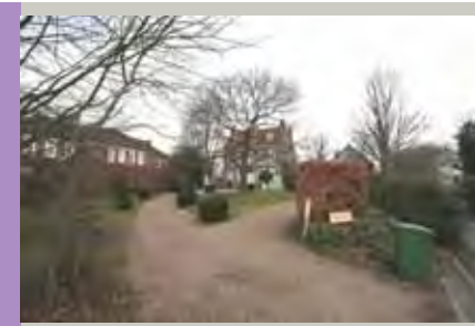
View of Manor House
