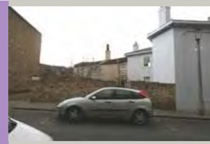
Wall between 1A and The Surgeons House
