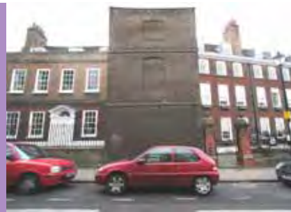
Wall between 12 and 14
