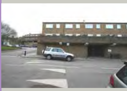
Rear of flats
