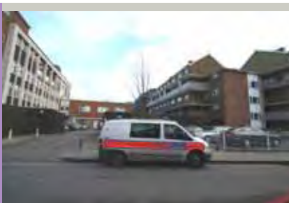
Maribor House / Police Station
