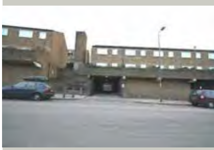
Rear of flats
