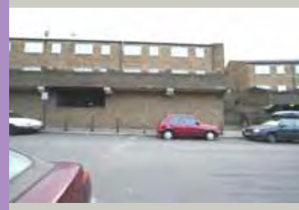
Rear of flats
