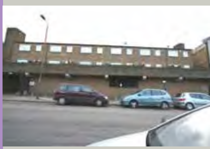
Rear of flats
