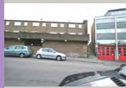
Rear of flats
