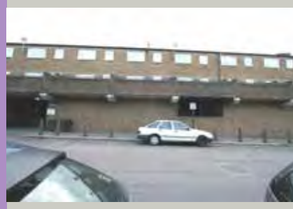
Rear of flats
