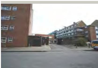
Maribor House / Police Station
