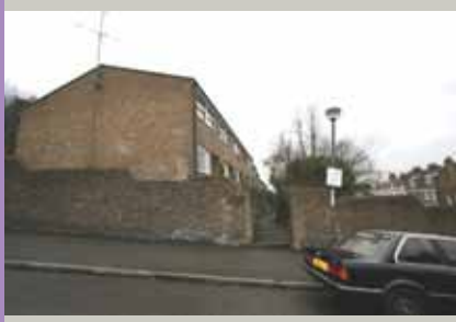
Wall and gable end
