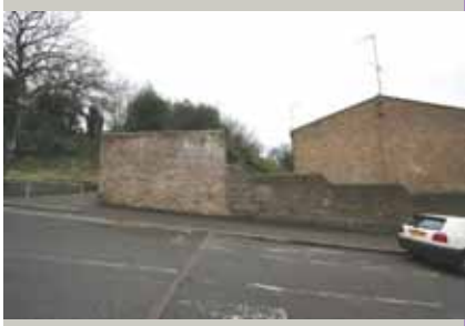
Wall and gable end
