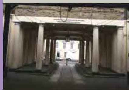
Greenwich Market north entrance
