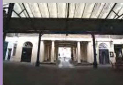
Greenwich Market north entrance
