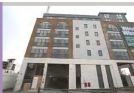
Wood Wharf, Horseferry Place (under construction)
