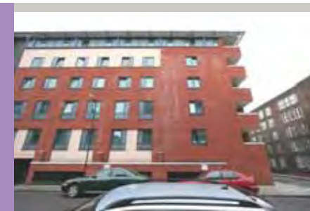
Flats and retail servicing
