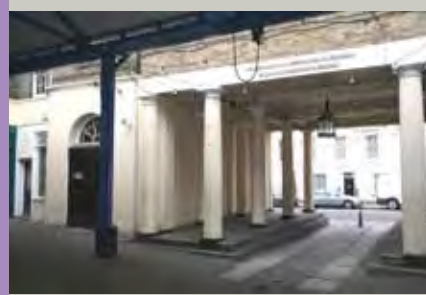
Greenwich Market north entrance
