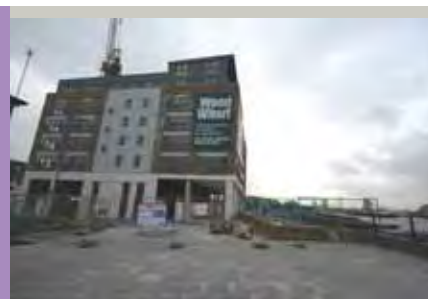
Wood Wharf, Horseferry Place (under construction)
