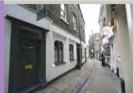
Oblique view west
