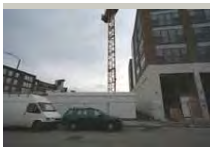
Wood Wharf, Horseferry Place (under construction)
