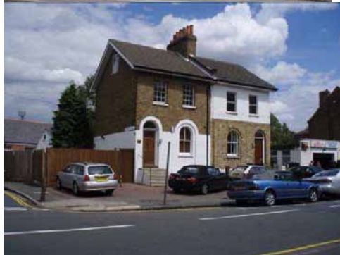
Figure 12: Charlton Road - gate post to demolished Eastcombe House - near corner of Sherington Road Figure 13: early Victorian 1840s style houses in 121-123 Old Dover Road
