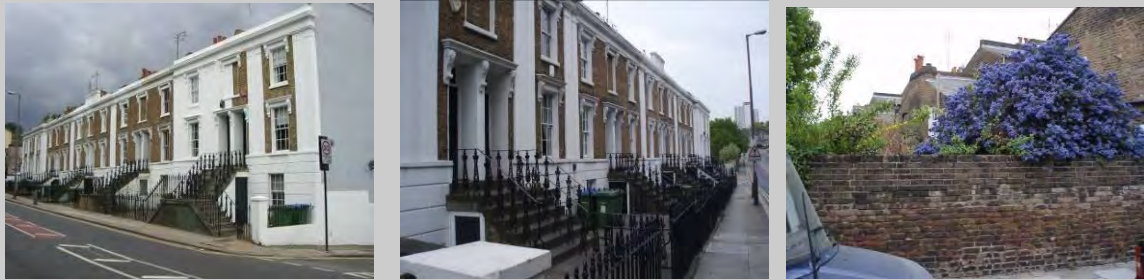
Figures 28 - 30: Former officer houses at 40-49 Hillreach & side wall to 49 Hillreach (in Woodhill).
