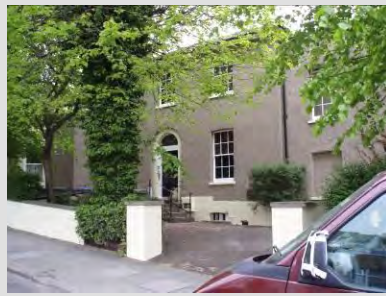
Figure 53: No. 98 (locally listed) double fronted with pebble dash over bricks and Georgian fanlight.
