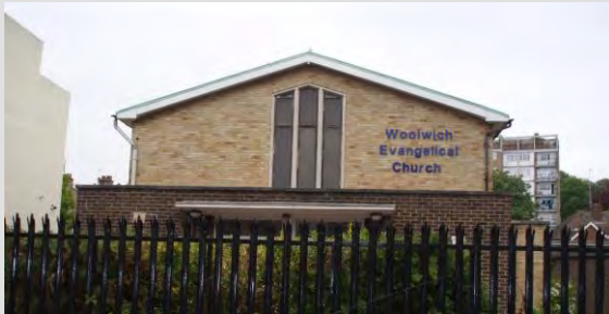
Figure 37: Woolwich Evangelical Church.
