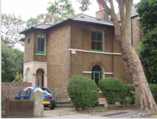
Figure 61: No. 70 Little Heath locally listed) and proposed to be added to the Conservation Area.
