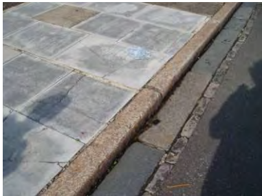
Figure 63: Red Lion Lane - granite channel and kerb outside Royal Military Academy.
