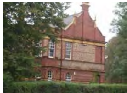
Figure 17: Victoria House - former Medical Officers Mess.
