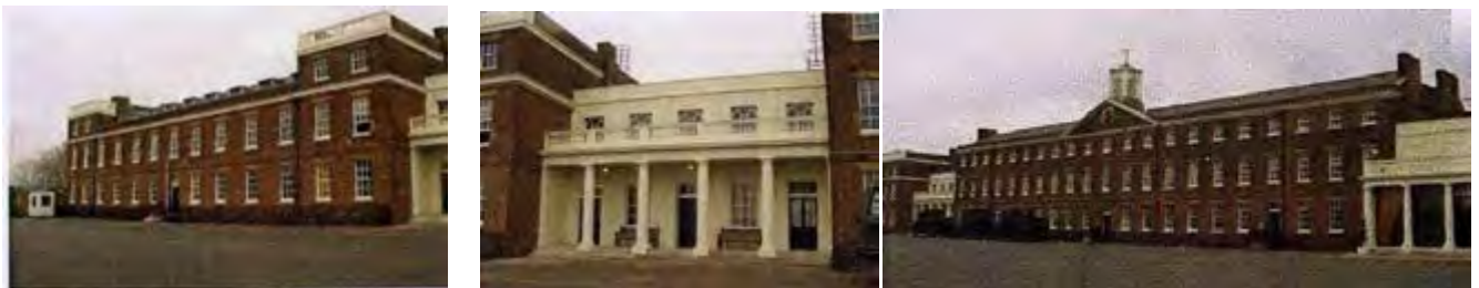
Figures 20 - 22: 1778 Barracks Buildings B1, B2 & B3.
