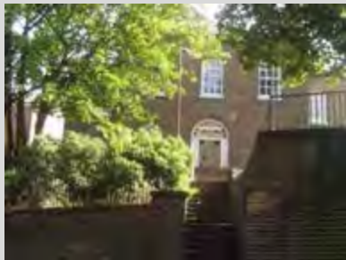
Figure 73: Engineer House – view from Woolwich New Road.
