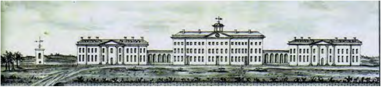
Figure 18: Sketch of Wyatt's late 18 th c Barracks by John Charnock, drawn c 1800, notice that there are now extra floors on the link blocks, towers at the ends of the wing pavilions, and minor changes to the roof. These changes can already be seen in the next picture from the early 19 th century.
