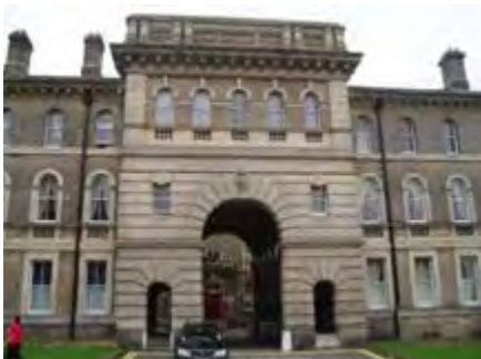
Figure 16: Herbert Hospital - main entrance block.
