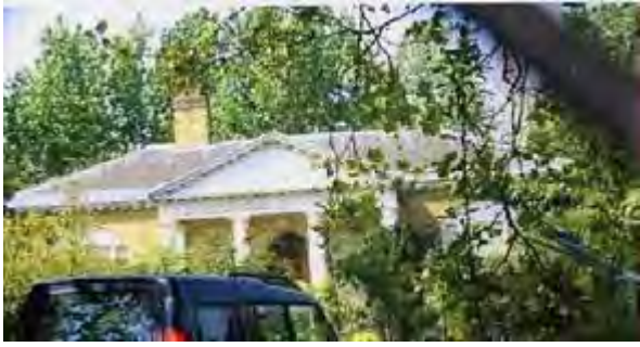
Figure 33: Former Commandant's house.
