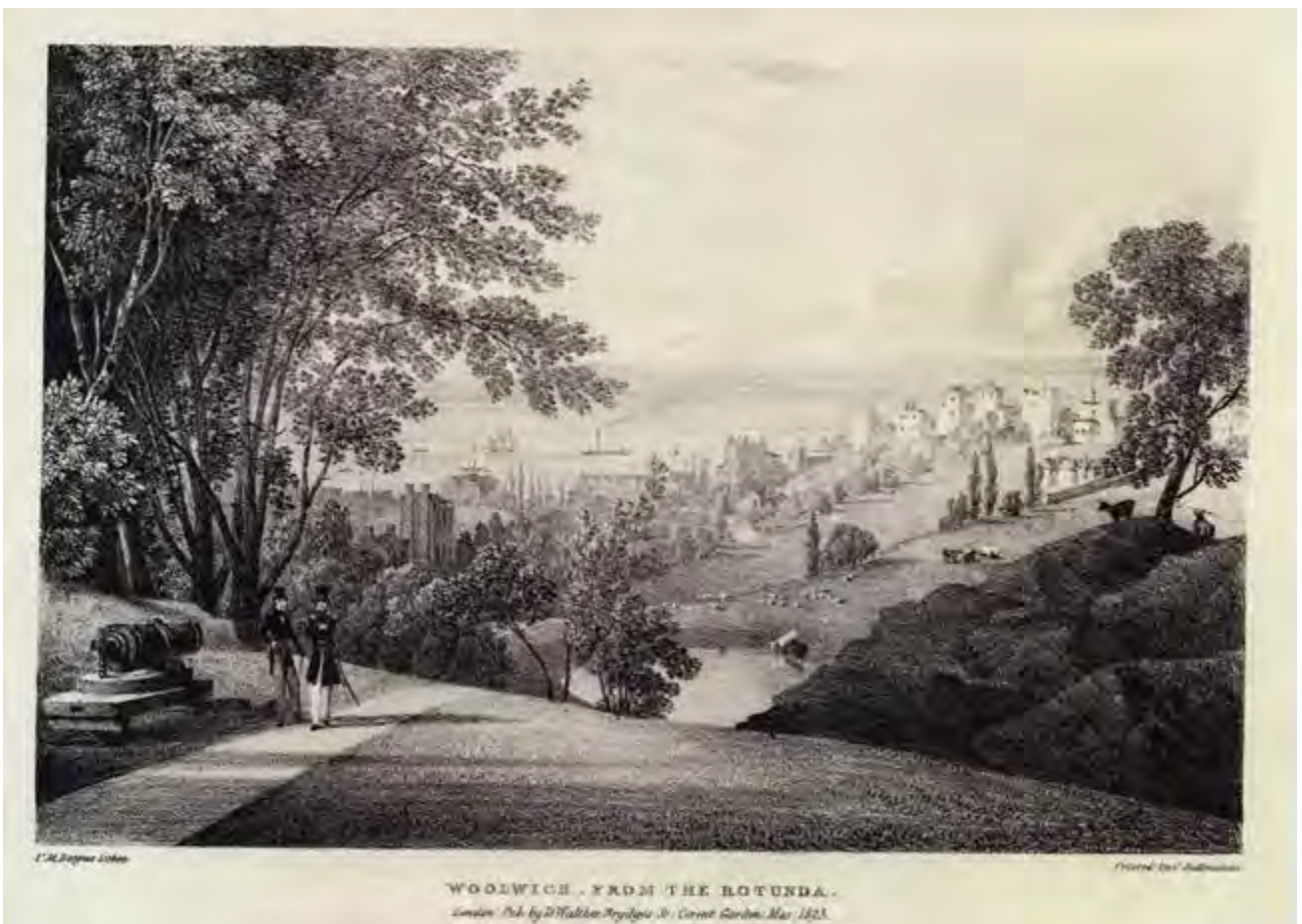
Figure 37: 1823 View from Rotunda, drawn three years after its relocation from Carlton House to Woolwich. Demonstrates hill-top location and fine views over old Woolwich and the river Thames. Note fix-mounted large Cannon in foreground.
