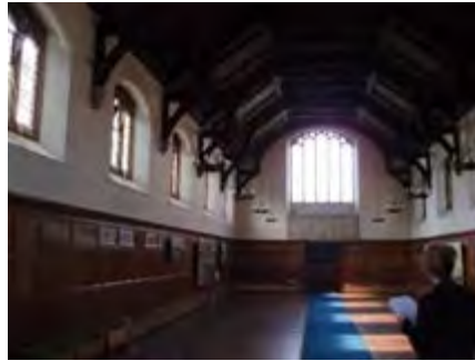
Figure 54: Church of St Michael and all Angels: interior with surviving hammerbeam roof.
