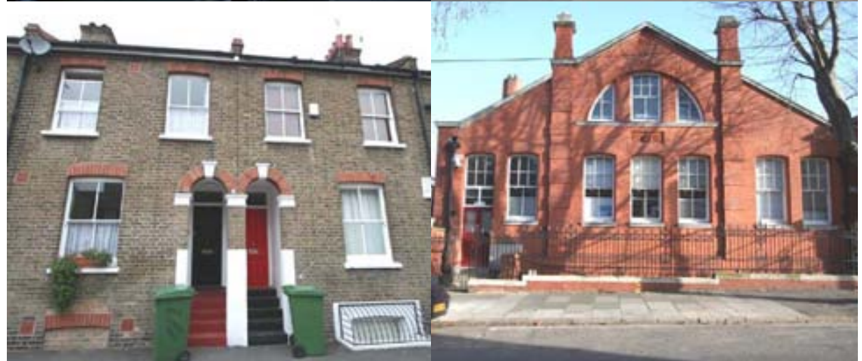
Top left: Trafalgar Road Top right: Late Georgian terrace, Old Woolwich Bottom left: Victorian terrace, Orlop Street Bottom right: Greenwich Primary Care Trust (1907), Greenwich Park Street
