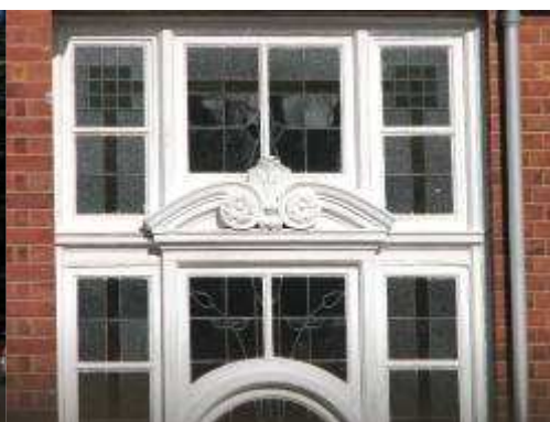
Detail of staircase window
