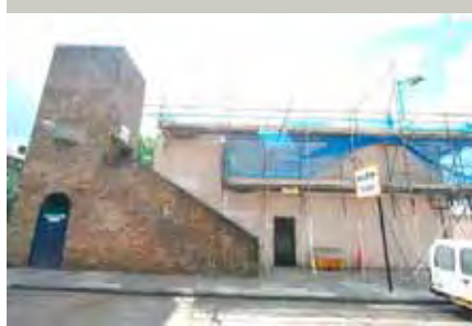
Side of 9-21 Combe Avenue
