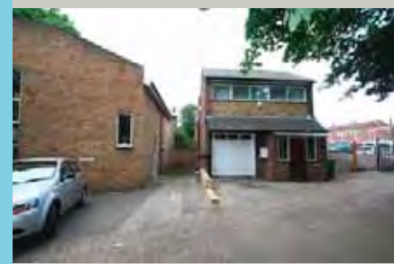
Rear of 1-10 Hatfield Court
