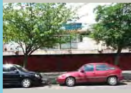
Rear of 9-21 Combe Avenue
