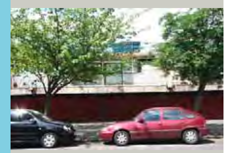
Rear of 9-21 Combe Avenue
