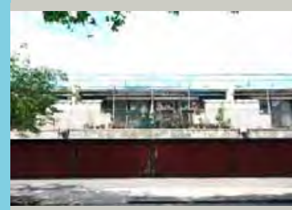
Rear of 9-21 Combe Avenue
