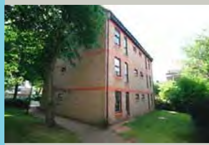
Rear of Park Road West
