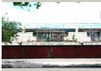
Rear of 9-21 Combe Avenue
