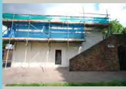
Side of 9-21 Combe Avenue
