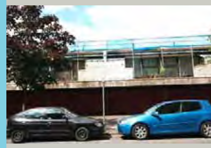
Rear of 9-21 Combe Avenue
