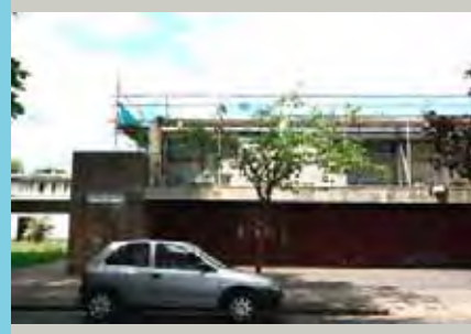
Rear of 9-21 Combe Avenue
