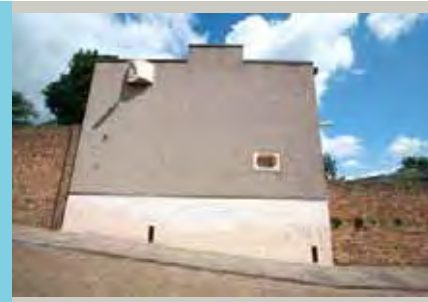
Side of 88 Combe Avenue
