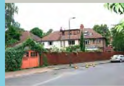
Rear of 98 Westcombe Park Road
