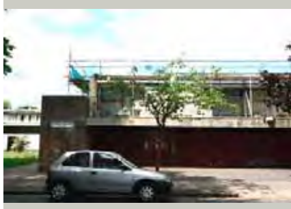
Rear of 9-21 Combe Avenue
