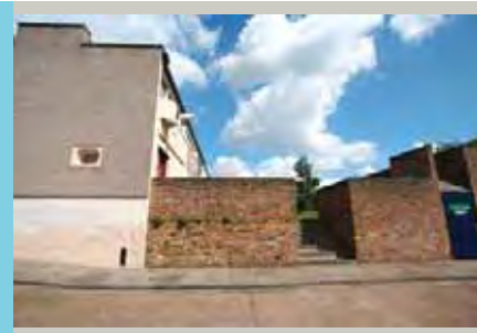
Side of 88 Combe Avenue
