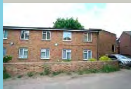
Rear of 1-10 Hatfield Court
