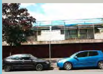
Rear of 9-21 Combe Avenue
