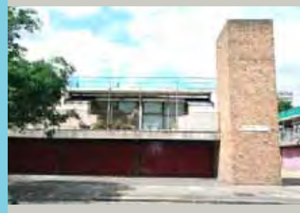
Rear of 9-21 Combe Avenue
