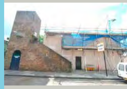
Side of 9-21 Combe Avenue
