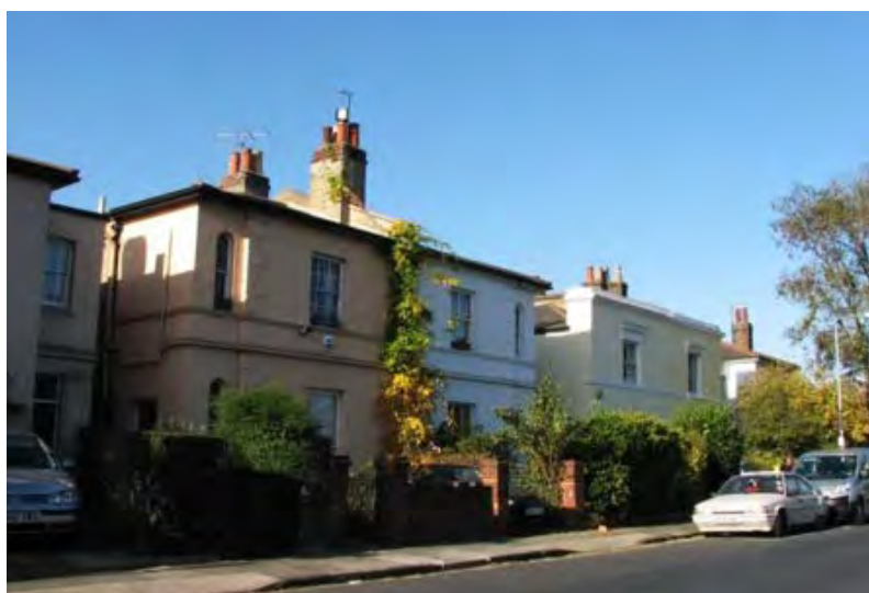
Figure 20: Grade II listed buildings on Fairfield Grove
