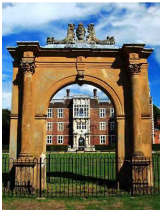
Figure 24: Former entrance archway
