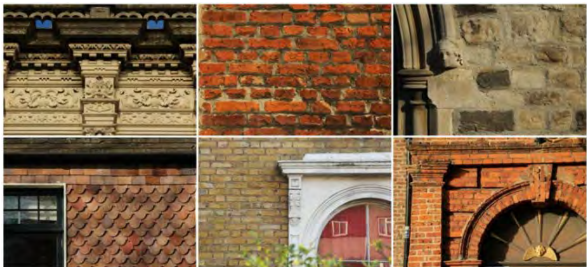
Figure 49: Clockwise from top left: Jacobean carved stonework; Jacobean red brickwork; mid-Victorian squared ragstone; mid-17th century moulded red brickwork; early-Victorian yellow stock brickwork and stucco window detailing; late-Victorian hanging tile
