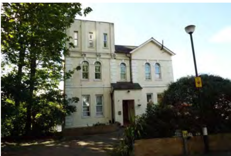
Figure 58: 87 Lansdowne Lane, a mid-19th century detached villa now divided into flats and largely stripped of its stucco ornament
