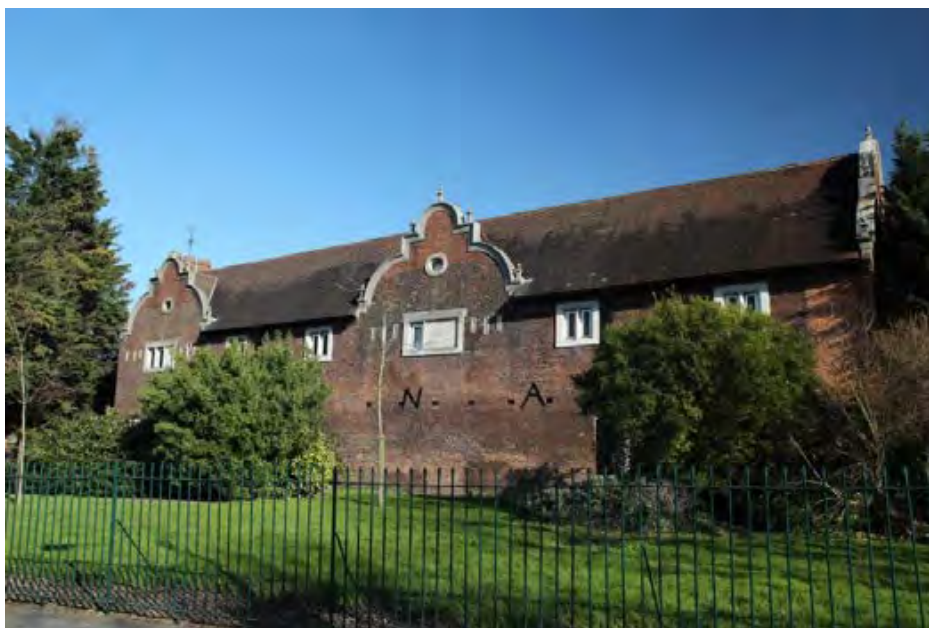
Figure 23: Stables: west wing
