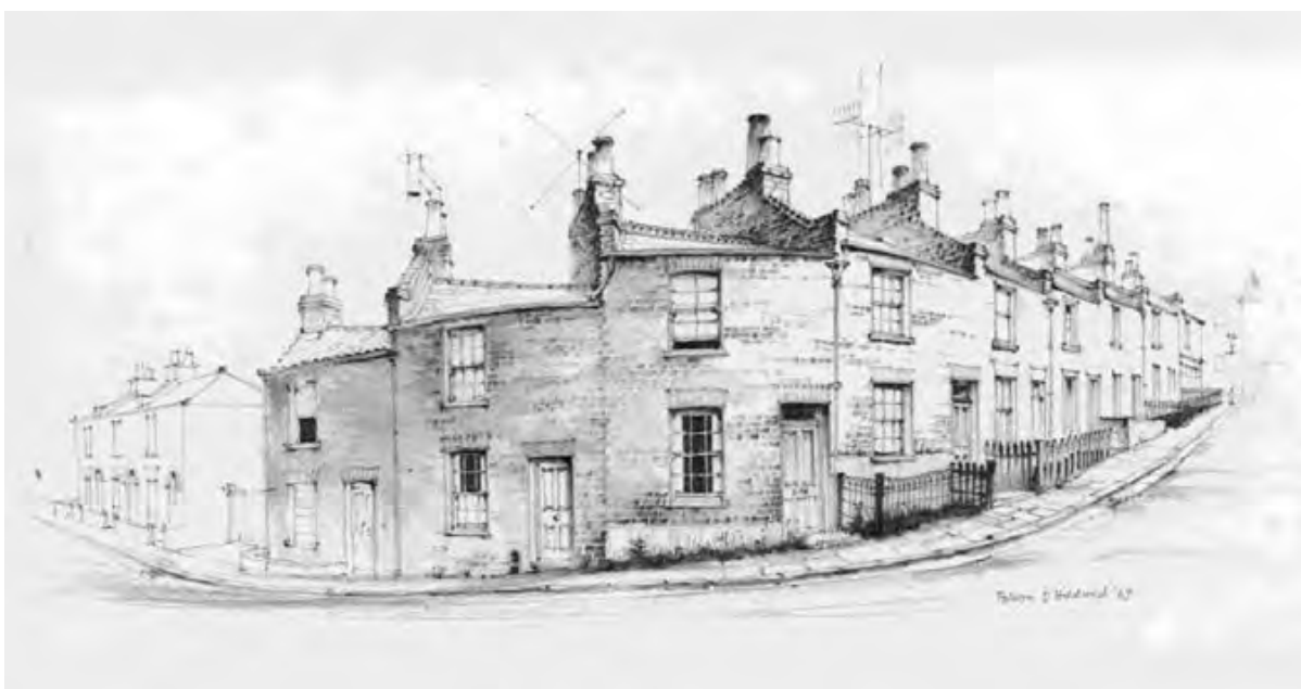
Figure 6: Nos. 2-18 Lansdowne Lane built 1862-3, drawn by Falcon Hildred in 1967 prior to their demolition in 1968 © Crown copyright: Royal Commission on the Ancient and Historical Monuments of Wales
