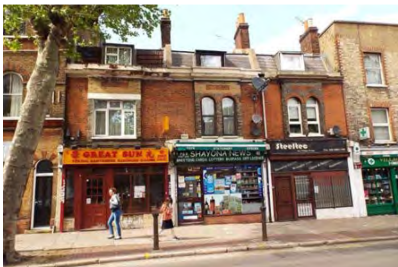
Figure 57: Replacement of shop-fronts, doors and windows in The Village
