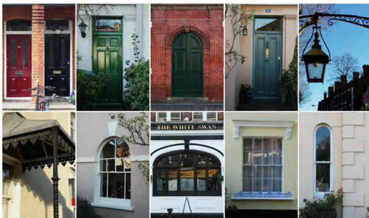
Figure 50: Examples of 19 th century panelled doors, decorative ironwork, sash and casement windows
