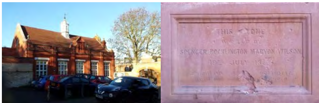
Figure 16: The Assembly Rooms, side elevation and foundation stone of 1886
