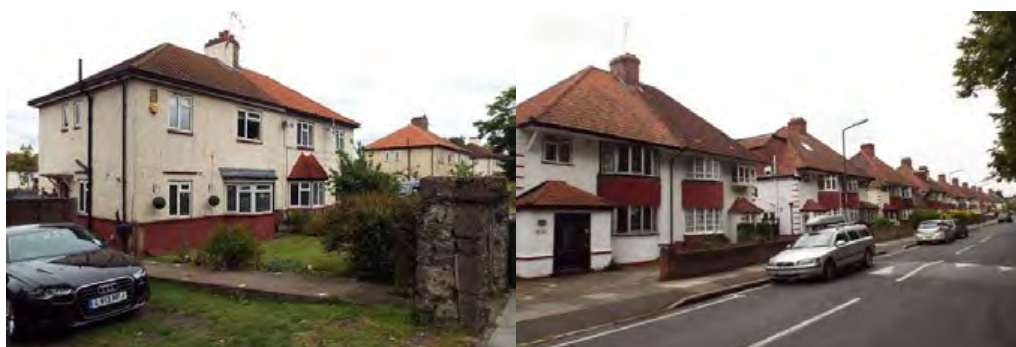
Figure 10: Houses in Charlton Park Road and Canberra Road
