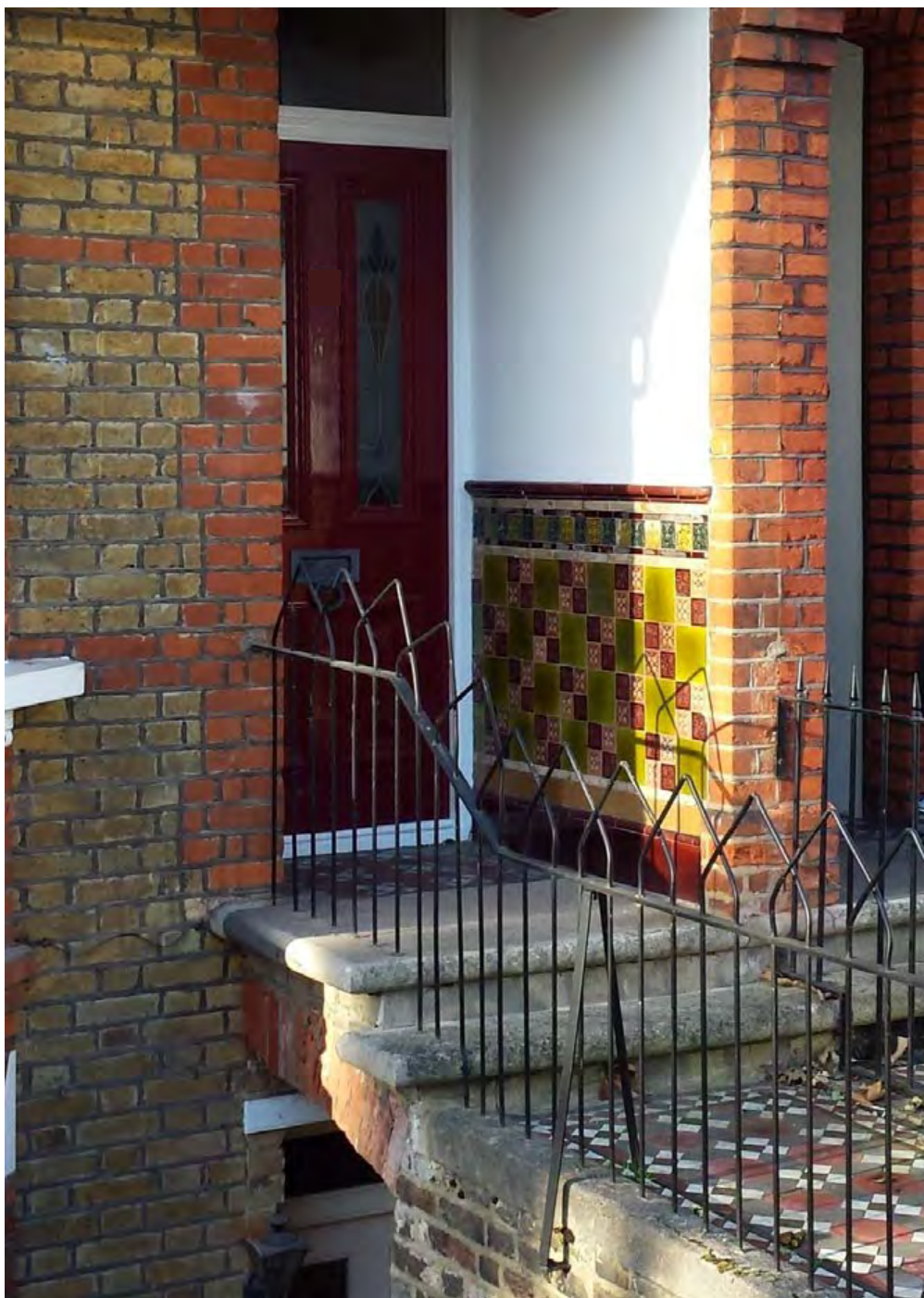
Figure 5: Lansdowne Lane: panelled door, decorative tiling and ironwork
