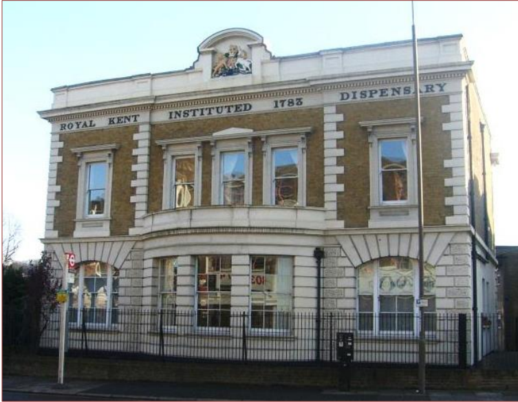
Figure 8: Mid-Victorian former dispensary building with stucco ornament
