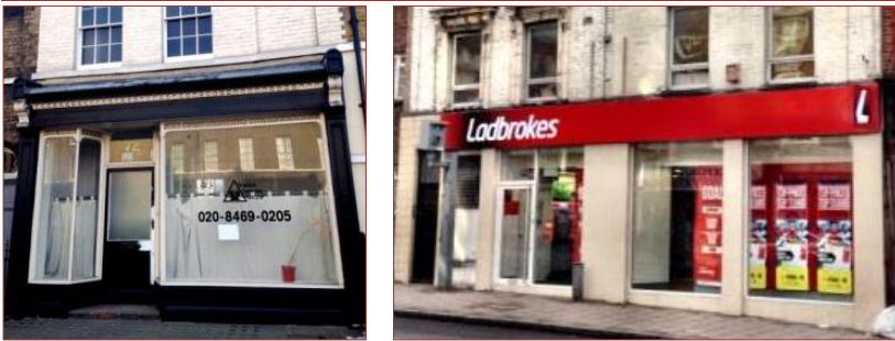
Figure 2: Historic shop front (l) and poor quality modern replacement (r)
