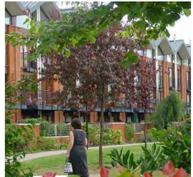
Town houses with apartments above (Coin Street)
