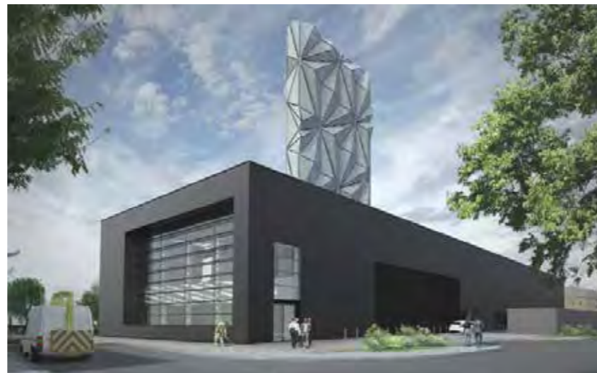
FIGURE 1.8 DISTRICT ENERGY CENTRE
