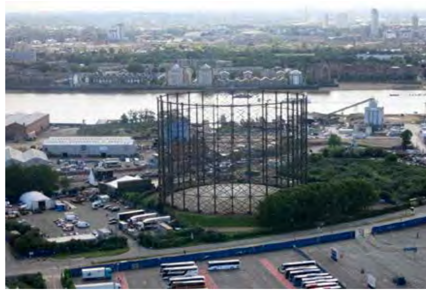
FIGURE 1.5 THE GAS HOLDER DOMINATES THE SKYLINE OF THE WESTERN GREENWICH PENINSULA
