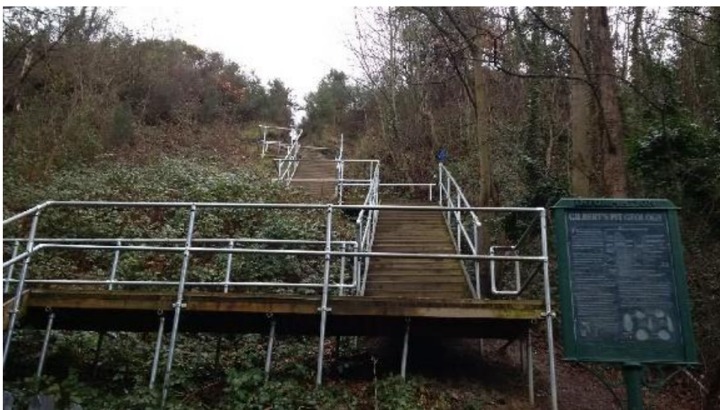
Stairway leading to Gilberts Pit.
