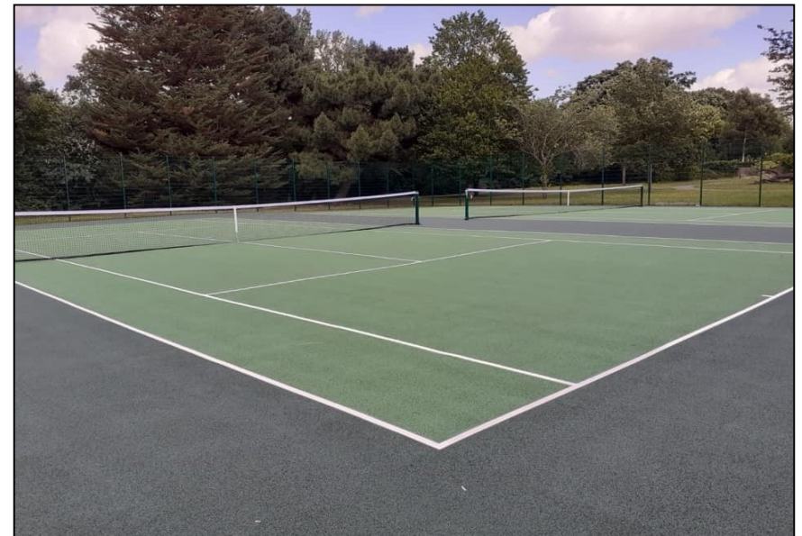
Resurfaced Tennis Courts
