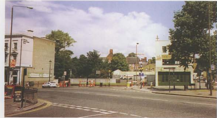
▲ Stockwell Street site: An important street junction where the building frontage needs to be re-defined by a strong architectural form
