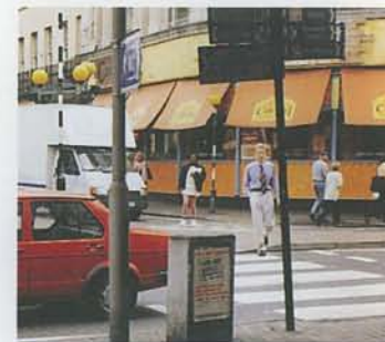
▲ A redundant control box and the base of an old lamp column now used as a support for pedestrian signing.
