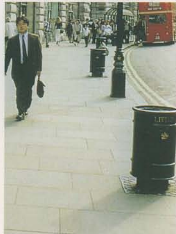
York stone paving and custom designed street furniture used in Regents Street. Note the use of grilles beneath the litter bins to prevent staining of the pavement by liquid waste.
