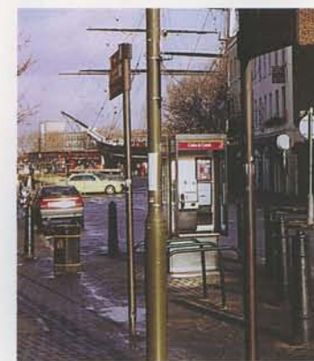
⚠ Visual clutter: Most of these posts and items of street furniture are either unnecessary or badly positioned.
