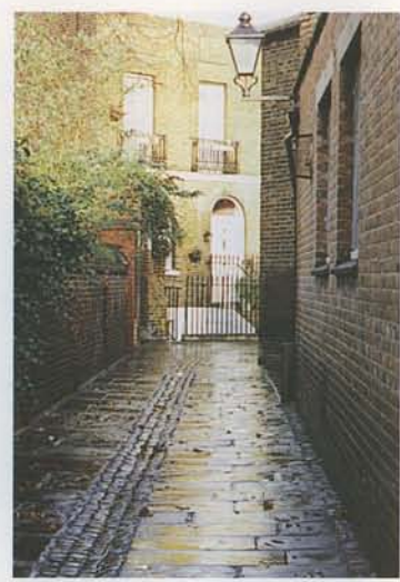
▲ St. Alfege Passage: Recently re-paved with York stone in a manner that is faithful to the original design.
