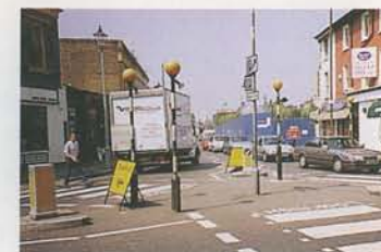
▲ Existing traffic island: showing a distinct lack of coherence.
