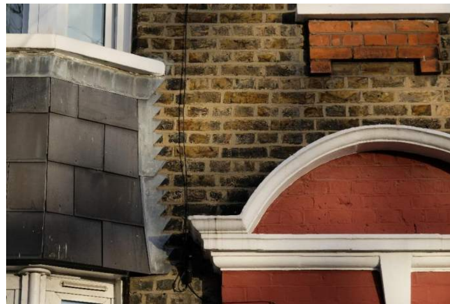
Riverside residential: Derrick Gardens, detail
