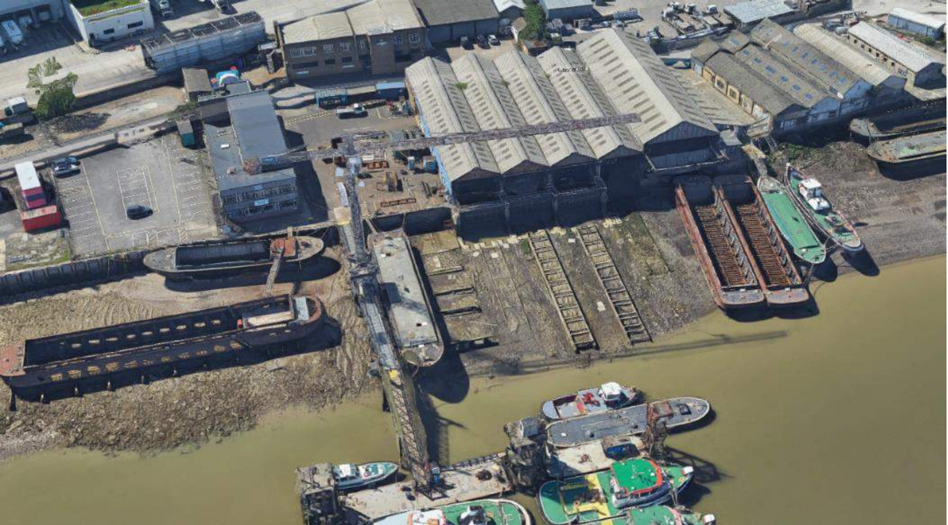
Cory's Barge Works from the north, showing boat repair sheds, covered slipways, office blocks, dry docks, slips, crane and jetty
