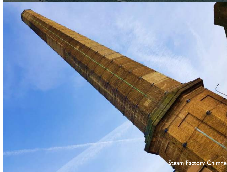
Steam Factory (former Erecting Shop, Brass Foundry and Smithery)
