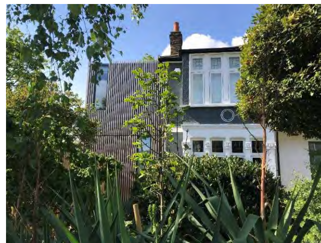
Right. Manor Park, Lee Forum area. Use of starkly contrasting geometry, materials and fenestration does not attempt to create an extension, rather an addition of the original house, from which the addition is clearly legible. Although the materials are not typical of the area, the use of timber softens the impact and fits in well with the mature landscaping and the riverside location. R2 Studio Architects
