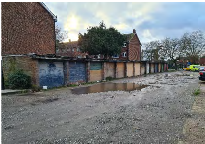
Garages off Burnt Ash Road, SA09
