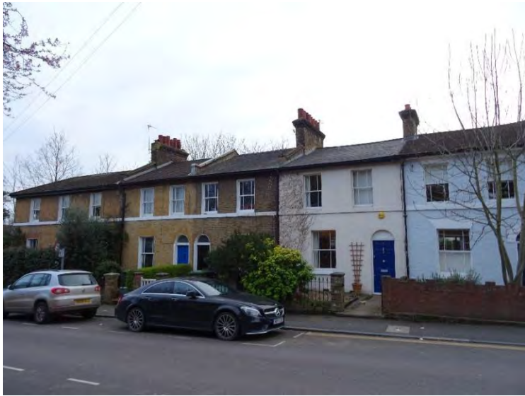
Surviving row of cottages in Dacre Park
