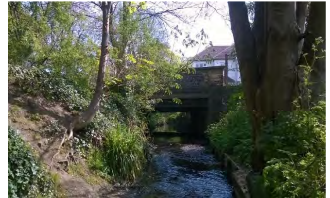
River Quaggy, Weigall Road bridge
