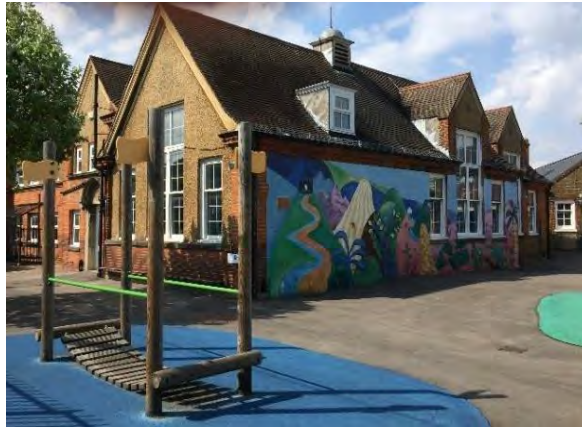
2. Community Infrastructure (Brindishe Lee School, Leahurst Road)
