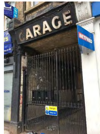
Old Garage Entrance, Lee High Road
