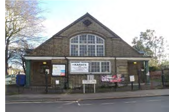
Grade II listed Lochaber Hall, one of several Community Centres
