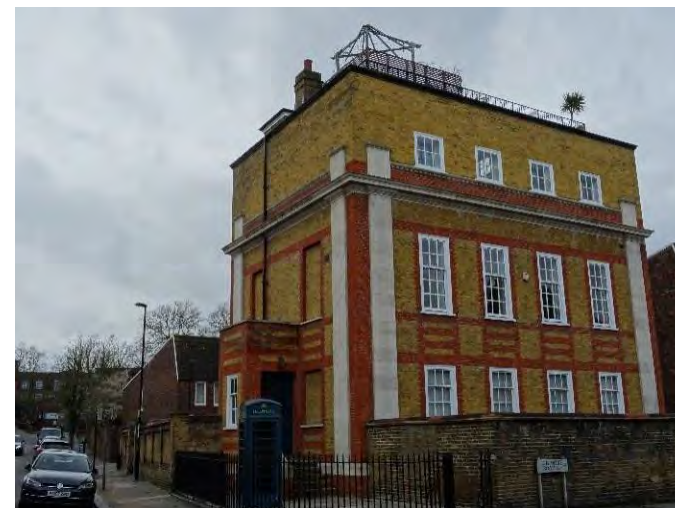
Above. cnr Gilmore Rd and Eastdown Park, Lee Forum area. Old Telephone Exchange. Grade II Listed building converted to residential whilst preserving the original external envelope. Blends contemporary elements such as glazed metal framed screens with original features. Flat roof has been transformed to a sun terrace. The Gilbert Scott designed telephone box previously stood outside the property, now stands next to the entrance housing a light sculpture.
