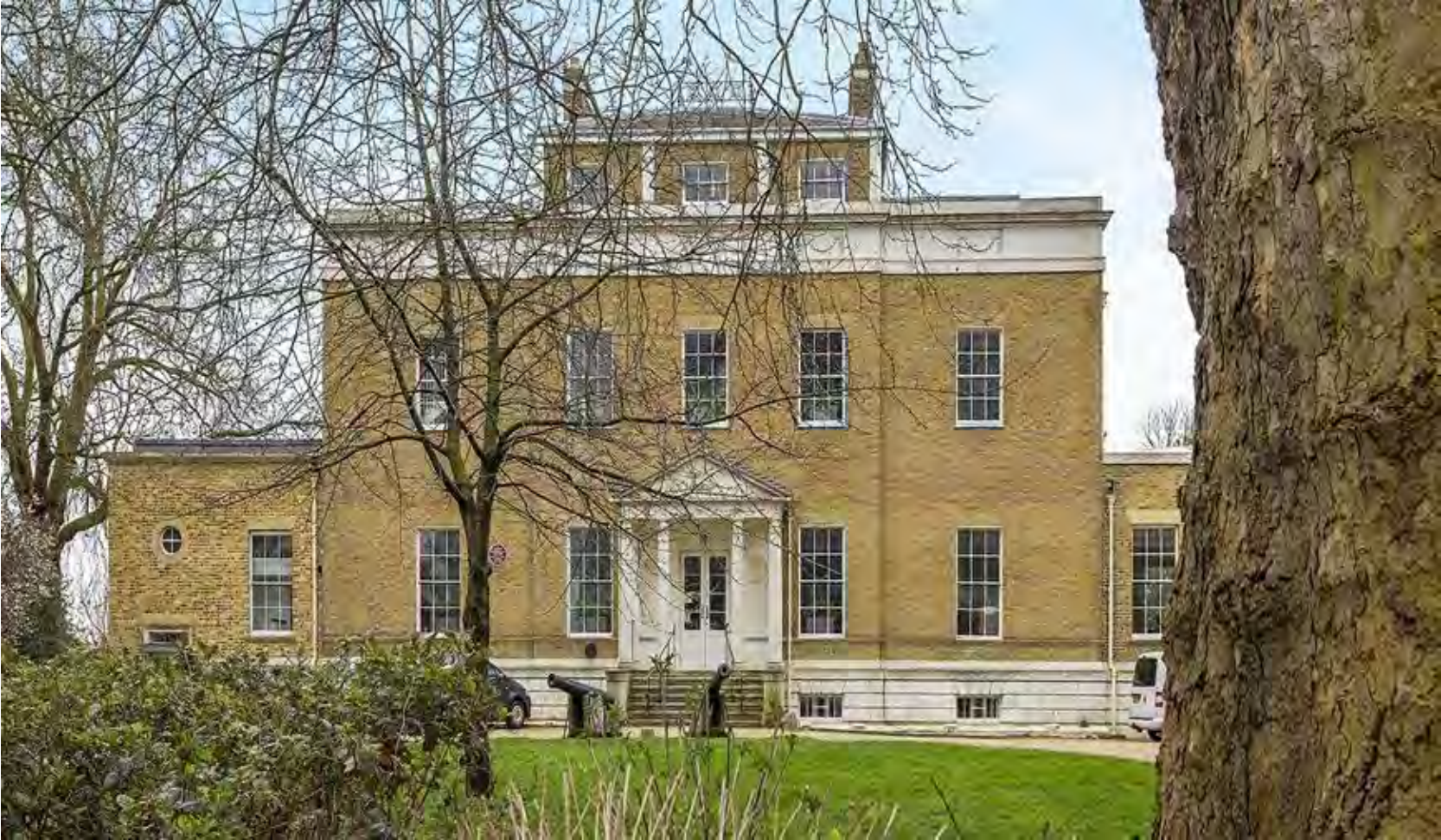
Grade II Listed Manor House, Old Road
