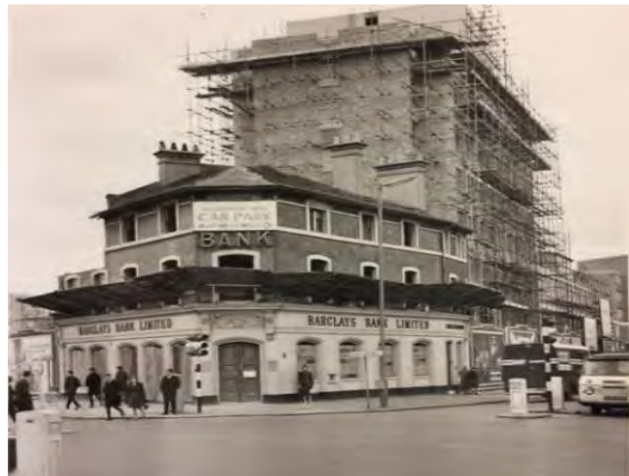
Lee Green Crossroads, towards Burnt Ash Road
