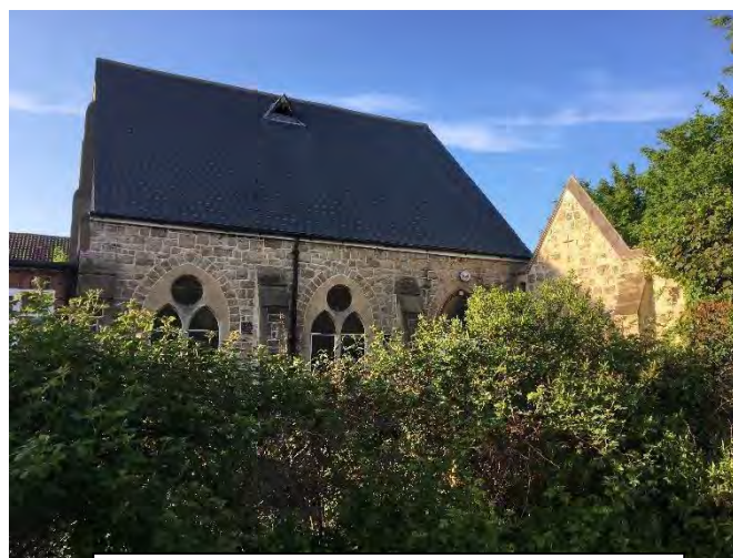
United Reformed Church, Burnt Ash Road
