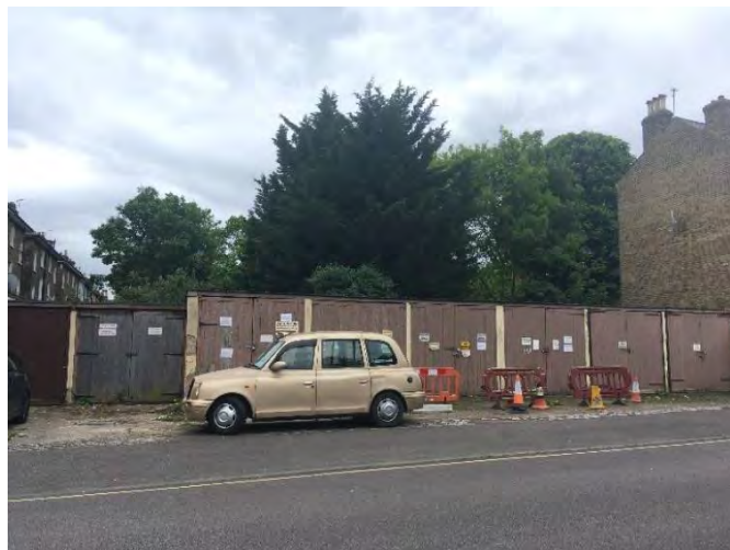
Garages, Wisteria Road, SA05
