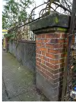
Bridge, Eastdown Park
