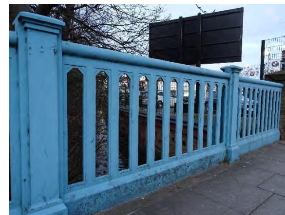
Bridge over River Quaggy, Lee High Road
