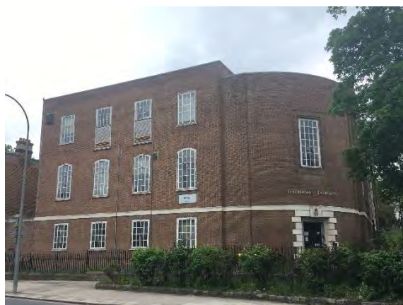
Telephone Exchange, Lee High Road
