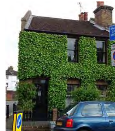
Hedgley Street/ Brightfield Road corner
