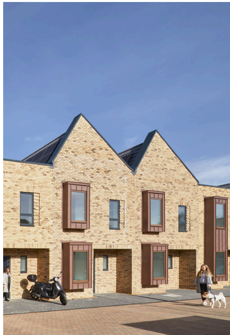
Underwood © Fuse Architects
