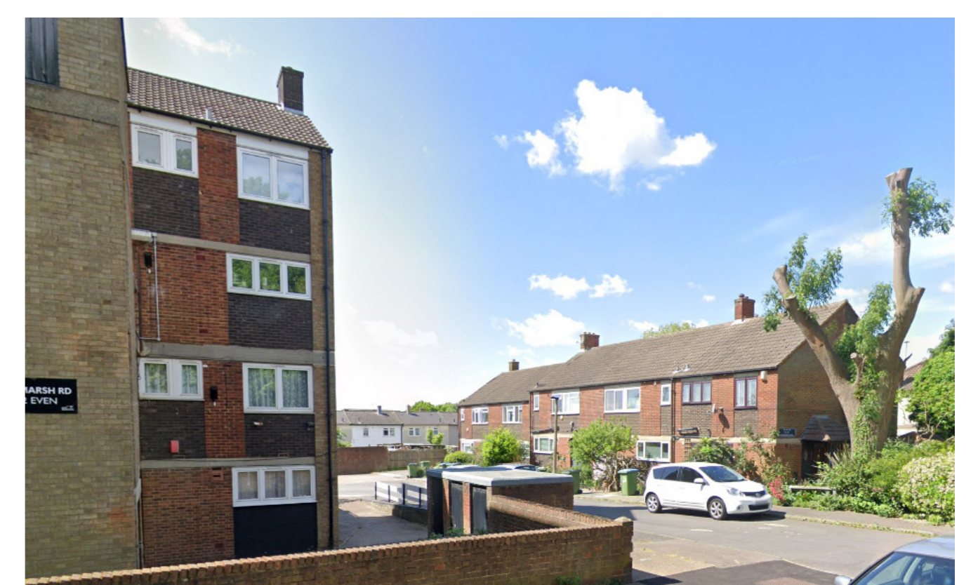
View looking south towards the Site from Wricklemarsh Road
